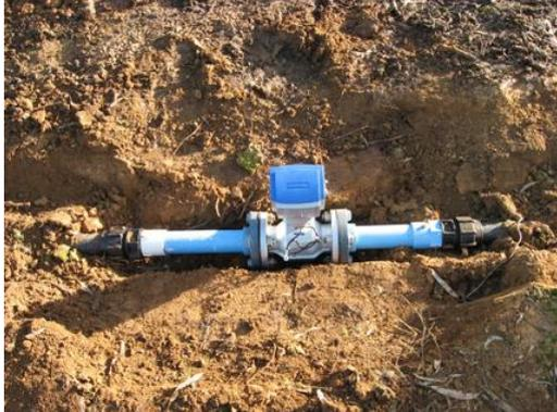
**Caption: WATERFLUX 3070 C installed in water pipeline**
